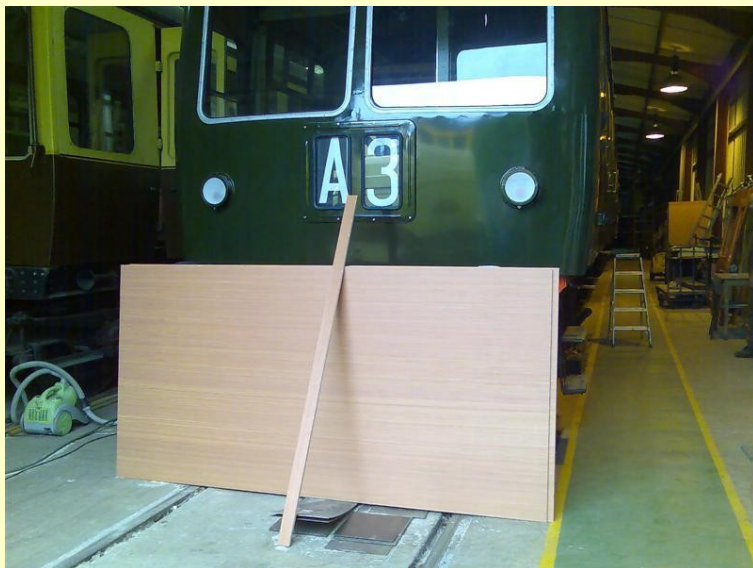
New flooring lined up for use inside 56456 (Llangollen Railcar Group)
